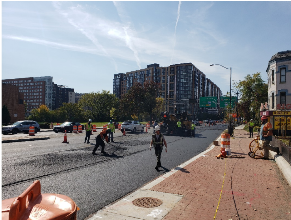
Picture No. 6 – 10/20/2020 – Installation of asphalt pavement in progress along NY Ave between NJ Ave and 4 th St. (West View)
