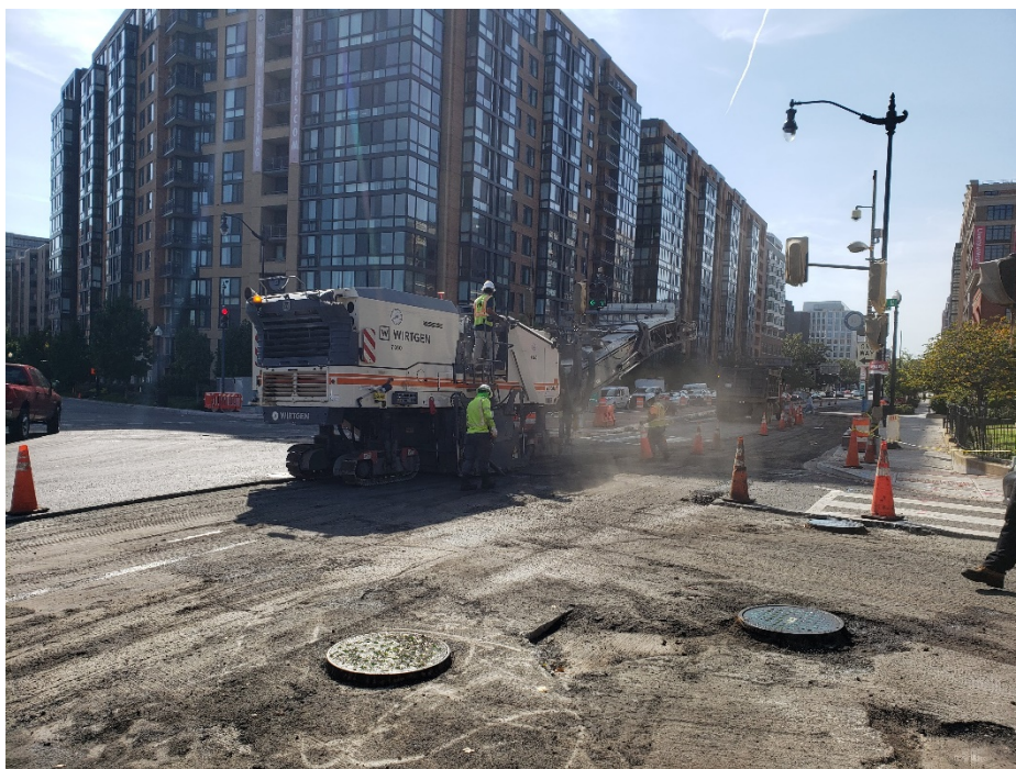
Picture No. 7 – 10/20/2020 – Pavement milling in progress along NY Ave and 4 th St. intersection (West View)
