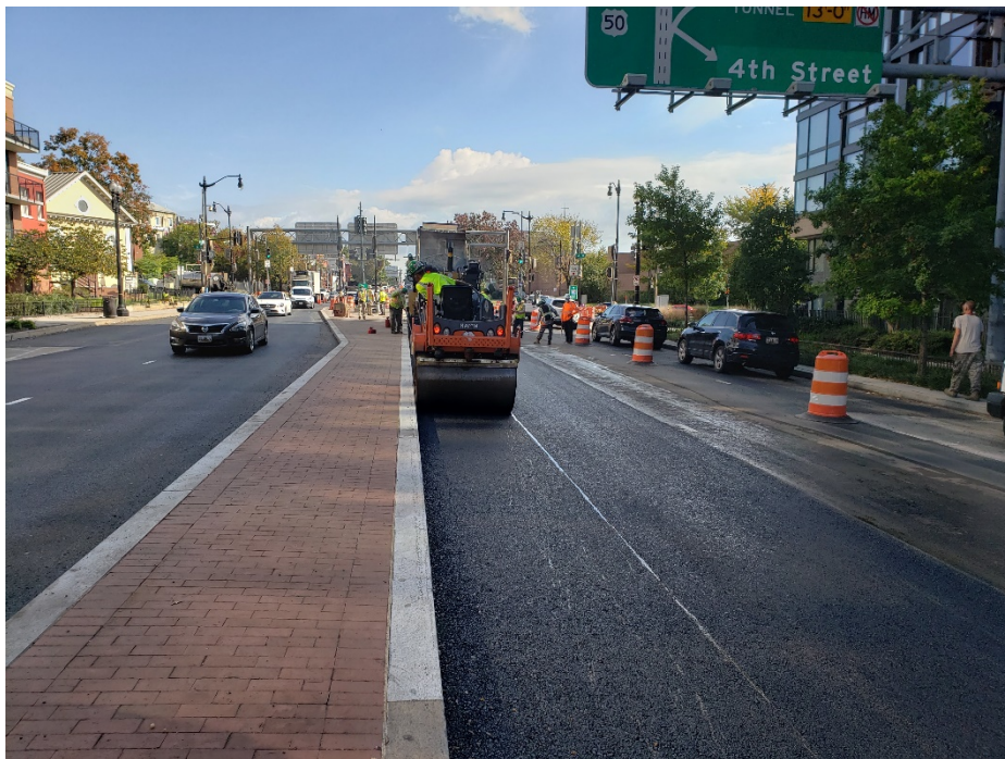
Picture No. 12 – 10/23/2020 – Asphalt pavement compaction in progress along NY Ave between 4 th St. and 5 th St. (East view)
