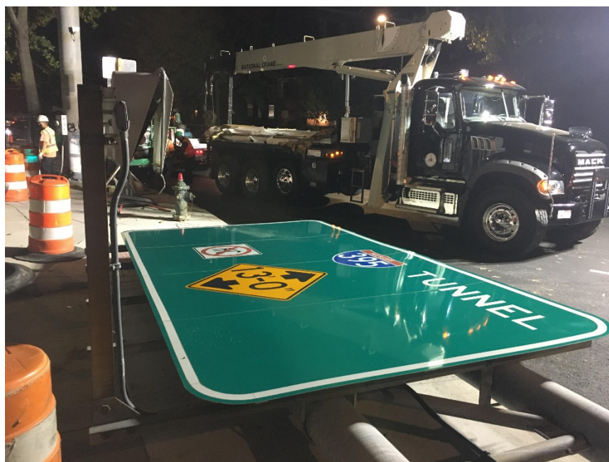
Picture No. 2: 10/18/2020 – Installation of overhead sign structure in progress along NY Ave and Kirby St. (East View)
