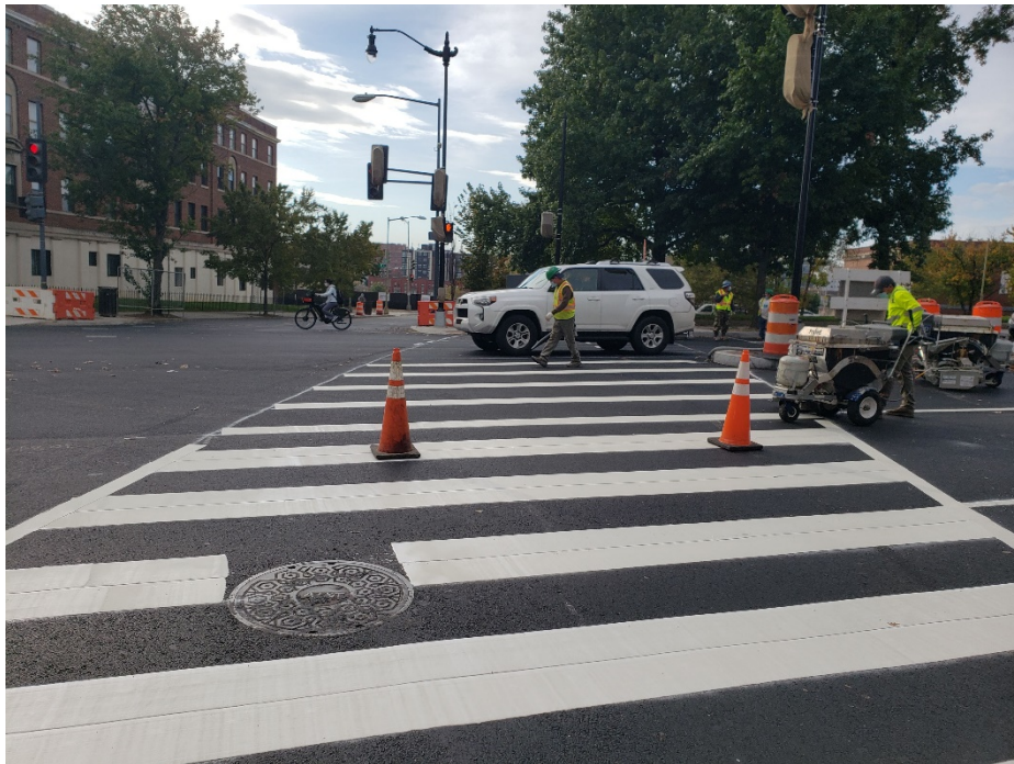
Picture No. 14 – 10/24/2020 – Line stripping in progress along NY Ave and 1 st St. (South view)
