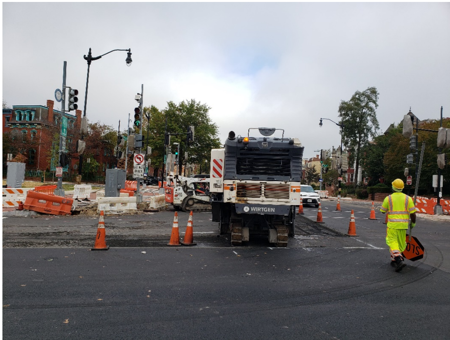
Picture No. 5 – 10/20/2020 – Pavement milling in progress along NY Ave and NJ Ave intersection (North View)
