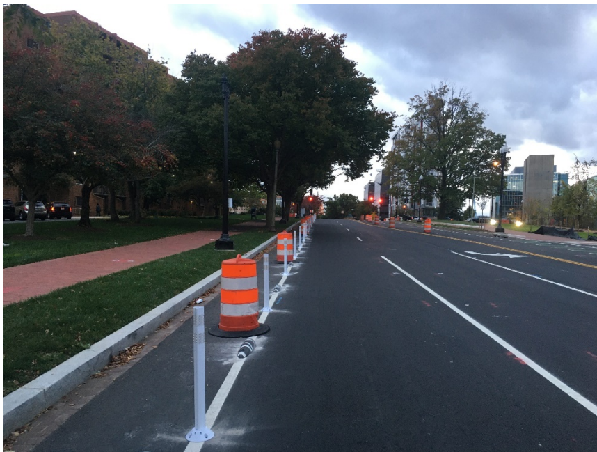
Picture No. 1: 10/18/2020 – Installation of delineators along NJ Ave between K St. and I St. (South View)
