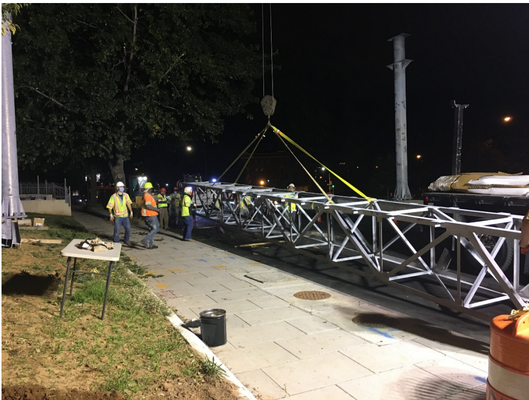
10/18/2020 – Installation of the overhead sign structure along NY Ave and Kirby St. (East View)
