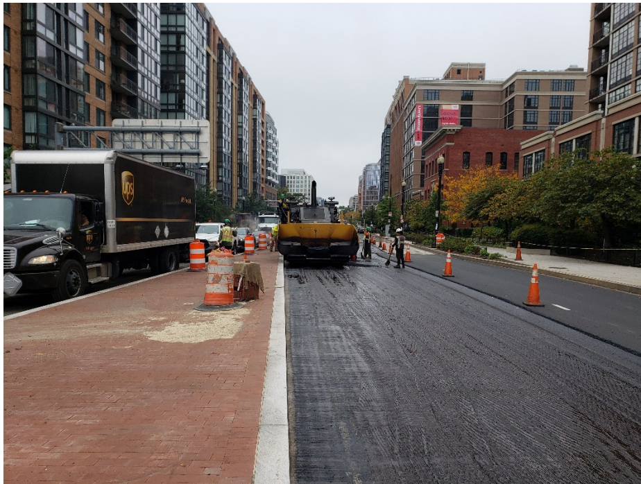
Picture No. 9 – 10/21/2020 – Tack Coat application along NY Ave between 4 th St. and 5 th St. (West view)
