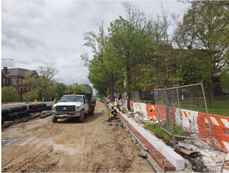
Picture No. 1: 04/27/2020 – Placing brick gutter at NY Ave. between 1st St. and Kirby St. WB. in progress along NY Ave between 1 st St. and Kirby St. (West View)
