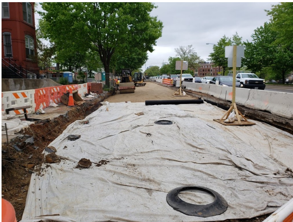
Picture No. 4 – 04/28/2020 – Placed plastic cover over exposed subgrade at NY Ave. between M St. and Kirby St. NB. (East View)
