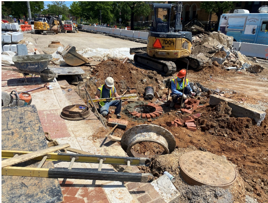
Picture No. 11 – 05/02/2020 – Adjustment of existing manhole near NY Ave. and M St (East view)
