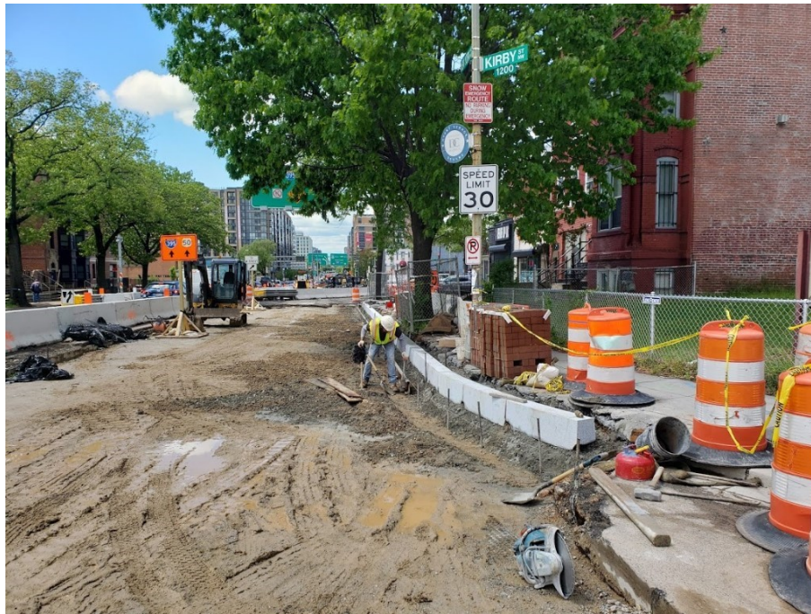
Picture No. 9 – 05/01/2020 – Furnished and installed granite curb at NY Ave. between M St. and Kirby St. NB. (East View)
