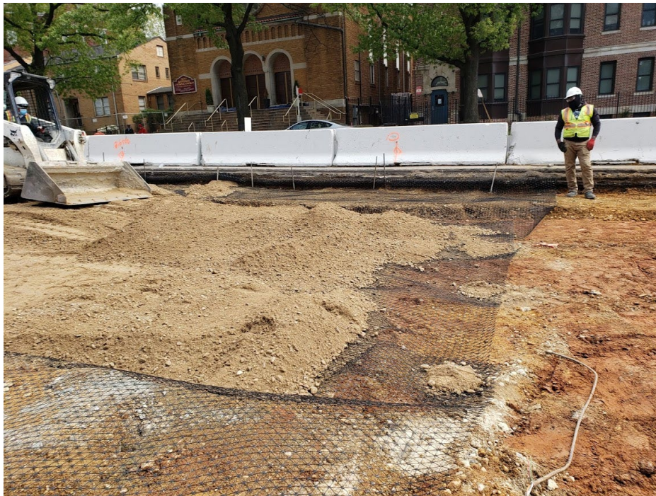
Picture No.7 - 04/29/2020 – Ongoing placement of TX7 Geogrid and aggregate base course at NY Ave. between M St. and NJ Ave. NB (South View)
