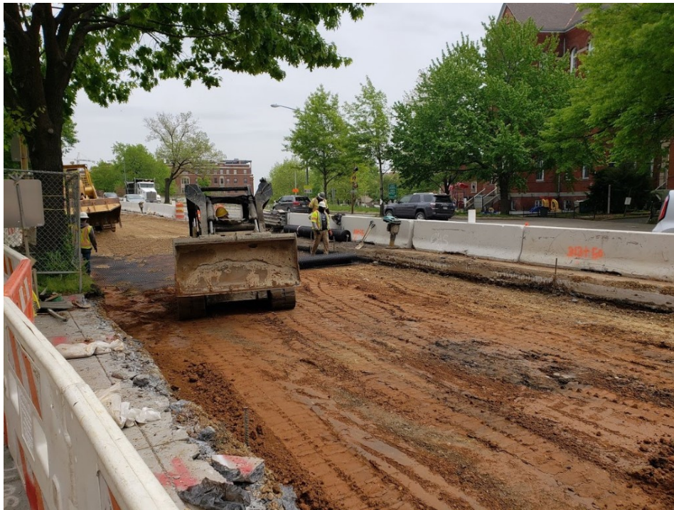
Picture No. 3 - 04/28/2020 – Grading, placing TX7 Geogrid and 21A stone at NY Ave. between M St. and Kirby St. NB. (East View)
