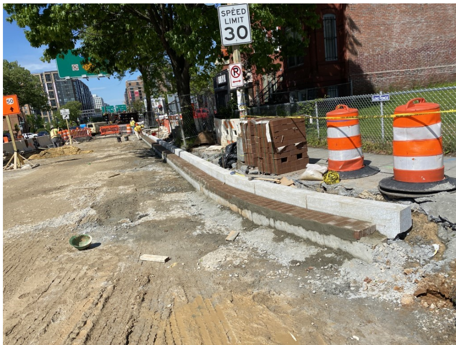
Picture No. 12 – 05/02/2020 – Brick gutter installation at NY Ave. between M St. and Kirby St. NB. (East View)
