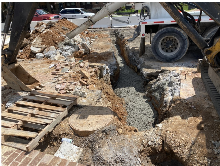
Picture No. 10 – 05/01/2020 – Conduit pipes encasement at NY Ave and M St. NW at NY Ave. and M St. NW (South view)
