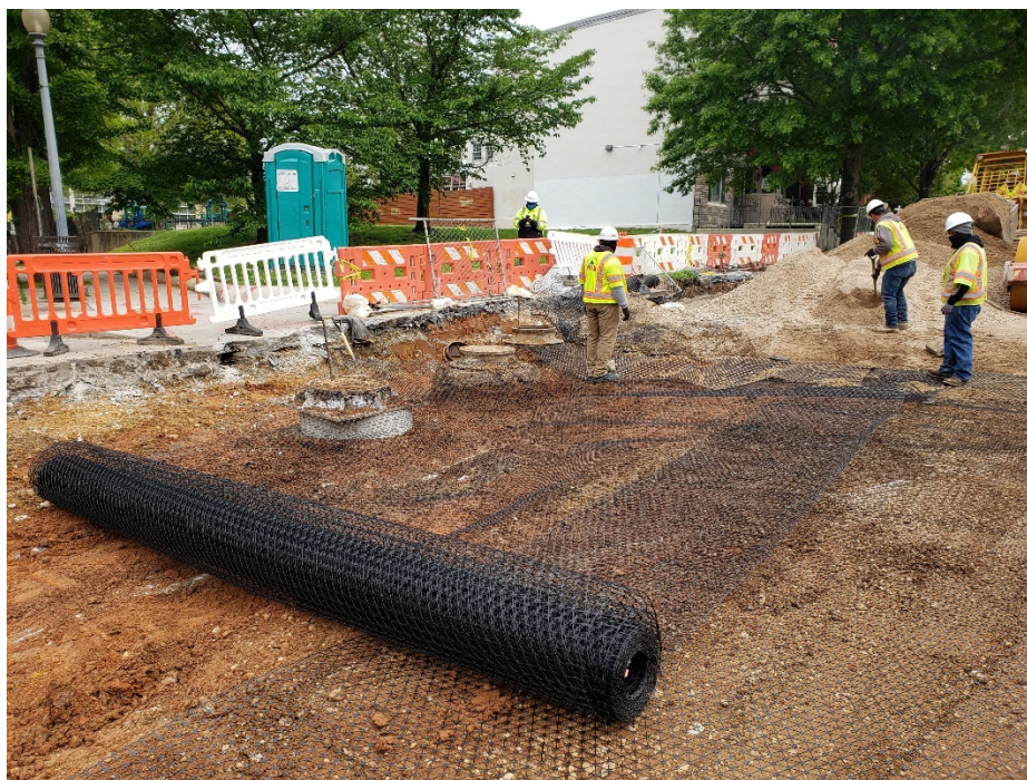
Picture No. 5 – 04/28/2020 – Grading and installation of TX7 Geogrid at WB NY Ave. NW at the intersection of Kirby St. (East View)
