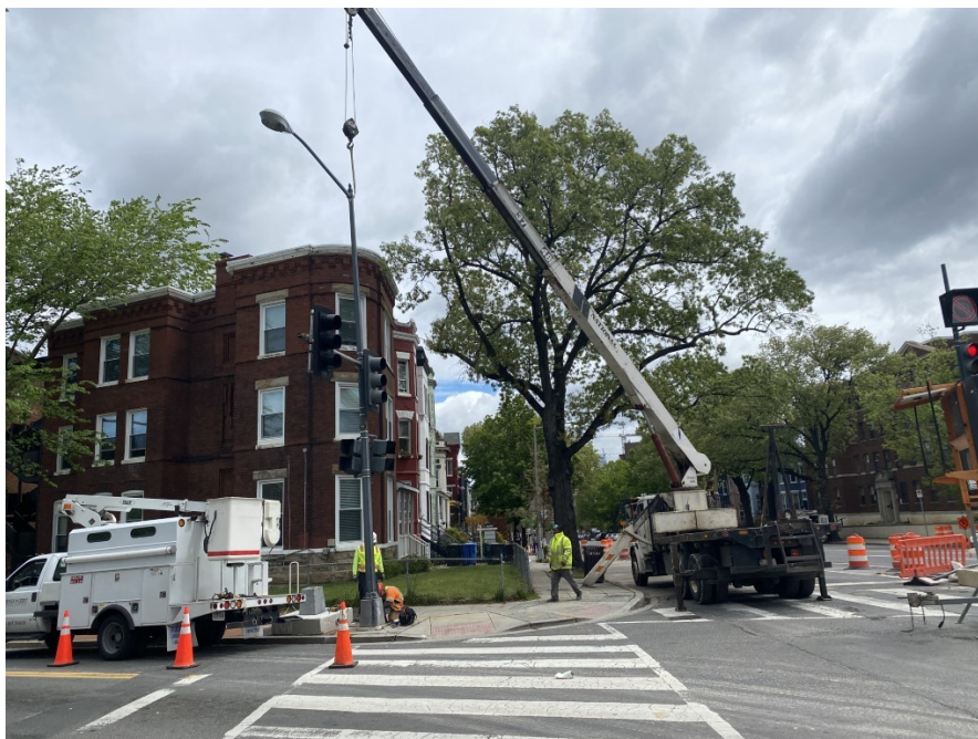
Picture No. 2: 04/27/2020 – Relocation traffic signal pole and equipment at the NY Ave. and 1st St. NW
