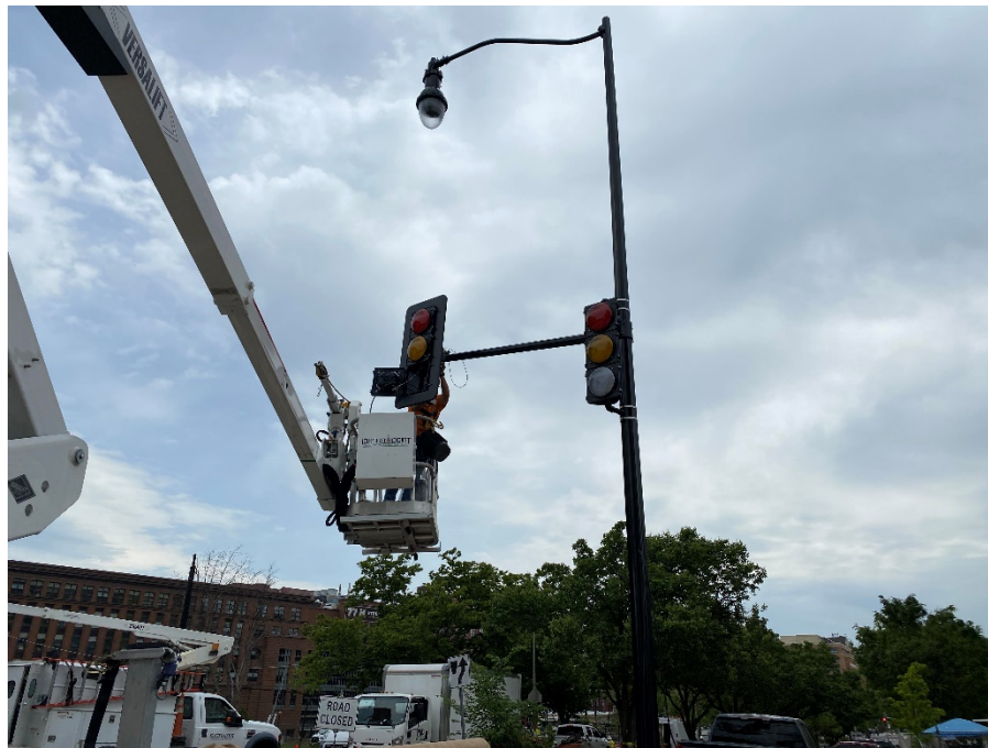
Picture No. 8 – 04/29/2020 – Installation of traffic signal equipment and streetlight fixtures at New Jersey and I Street NW (South view)
