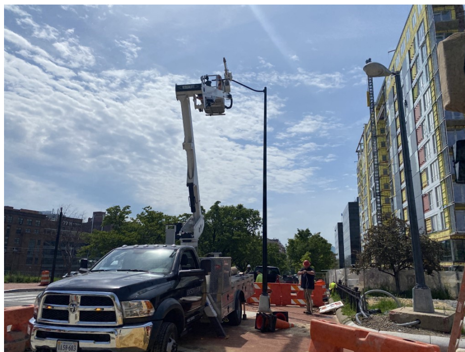
Picture No. 6 – 04/29/2020 – Installation of traffic signal equipment and streetlight fixtures at New Jersey and I Street NW (South view)
