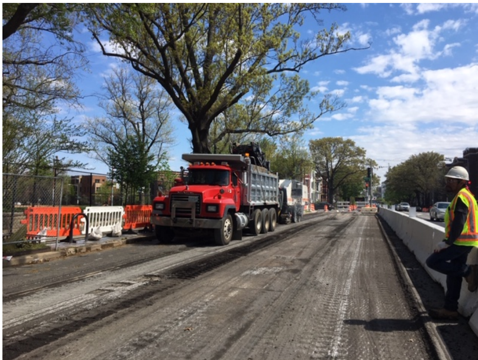
04/14/2020 – Pavement milling along westbound NY Ave between 1 st St. and Kirby St. (East View)
