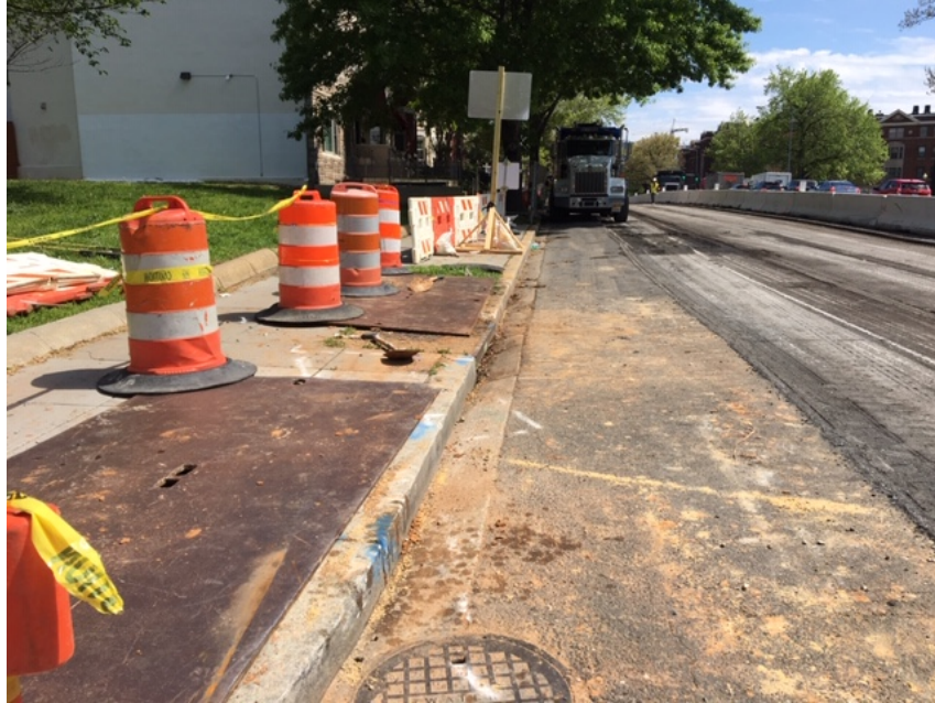
Picture No. 1: 04/14/2020 – Hard surface excavation (pavement milling) in progress along NY Ave between 1 st St. and Kirby St. (East View)
