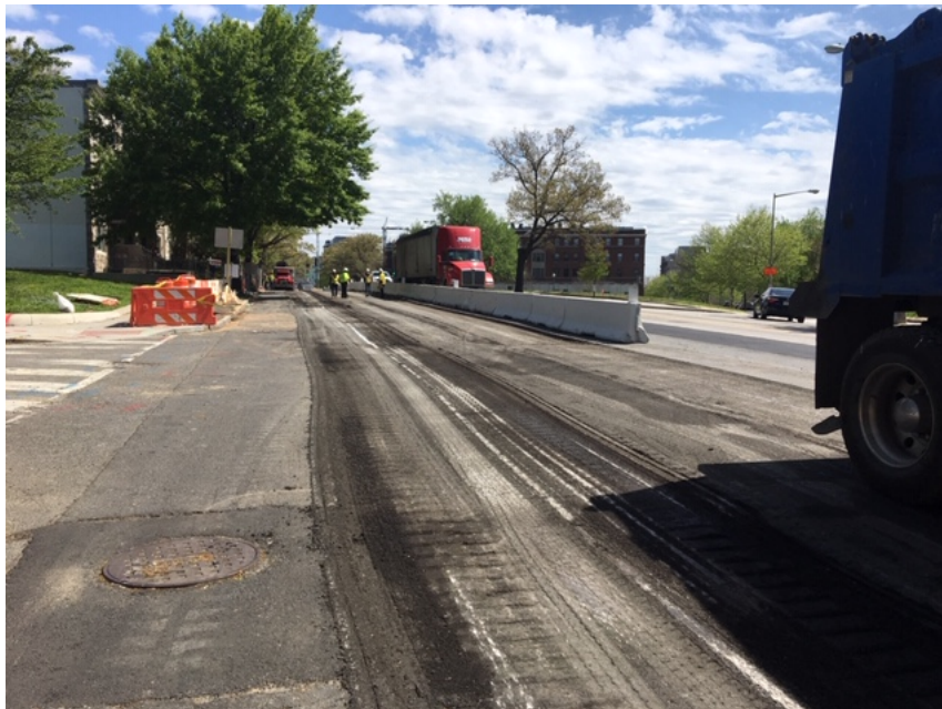
Picture No. 2: 04/14/2020 – Hard surface excavation (pavement milling) in progress along NJ Ave between 1 st St. and Kirby St. (East View)
