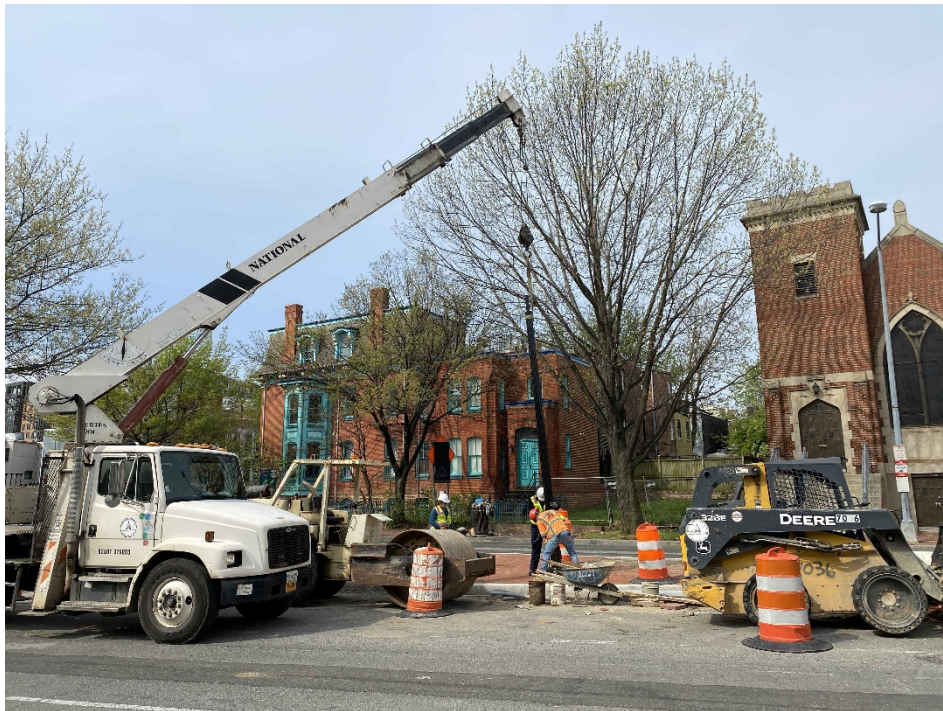
Picture No. 7 - 04/17/2020 – Installation of streetlight pole at the island along NJ Ave between M St. and Morgan St. (West View)
