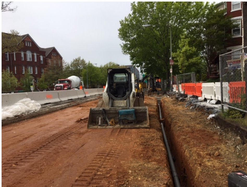
Picture No. 6 – 04/17/2020 – Installation of PVC conduit along NY Ave between 1 st St. and Kirby St. (West View)
