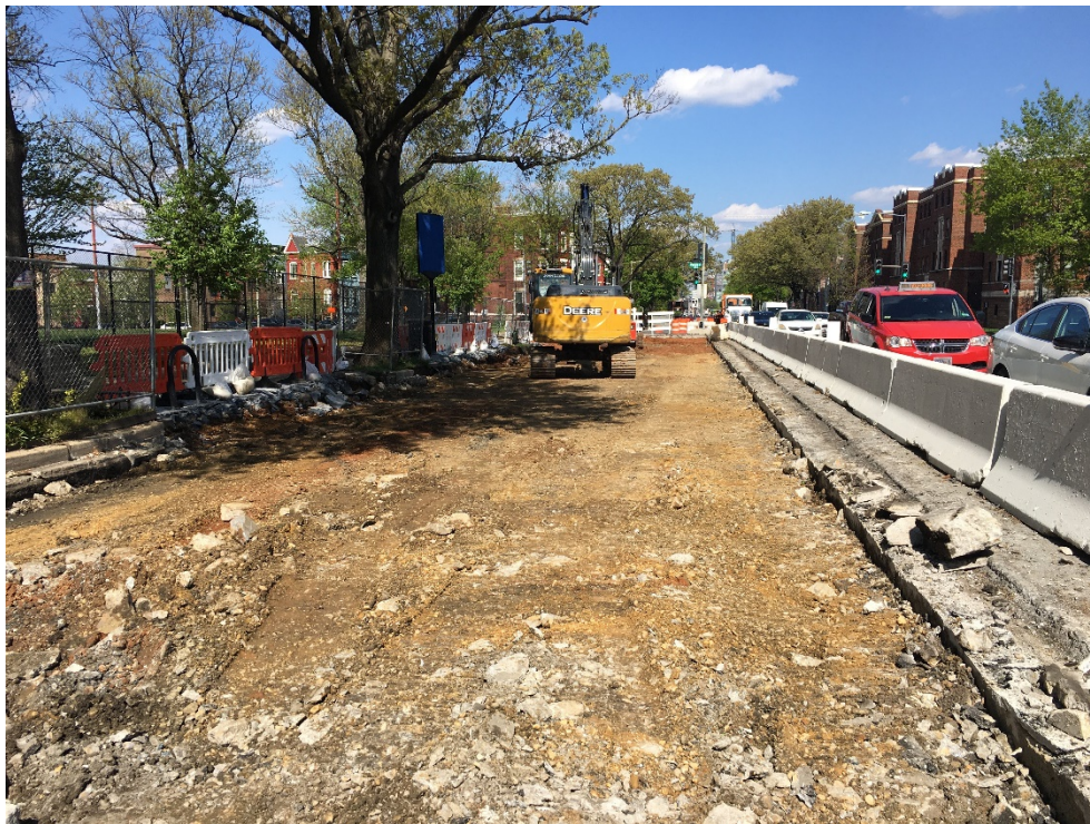
Picture No. 4 – 04/15/2020 – Full depth excavation at the intersection of NY Ave and 1 st St. (East View)
