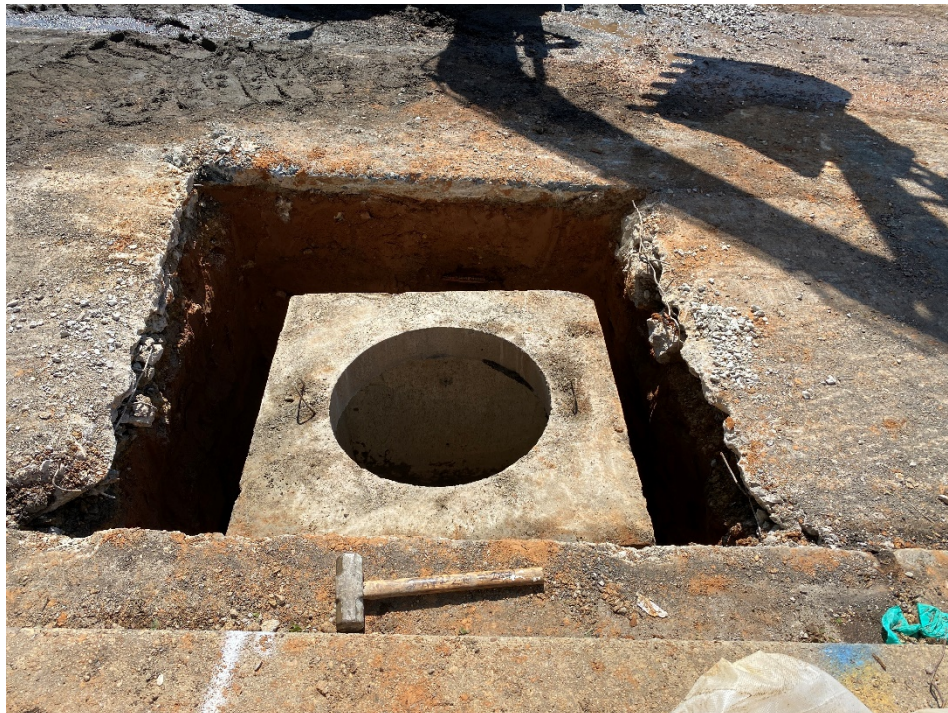
Picture No. 5 – 04/15/2020 – Installation of 36" x 36" manhole along NY Ave at the intersection of NY Ave and Kirby St. (South View)
