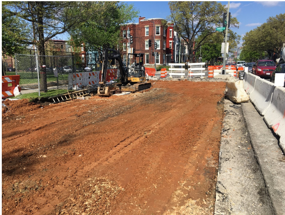
Picture No. 3 - 04/15/2020 – Full depth excavation at the intersection of NY Ave and 1 st St. (East View)
